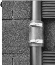
**Important:** If installing on a roof, use a silicone sealant to prevent water leakage into structure. Apply adequate amounts of sealant to both the pre-drilled hole and over the screw head on
