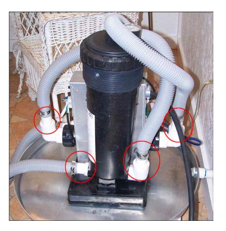
The side picture shows a leaking pump and filter assembly. We have circled the hose connections in this picture. There are two more not visible in this picture that are connected the same way. The leaks are a result of the hoses not being on fully.
